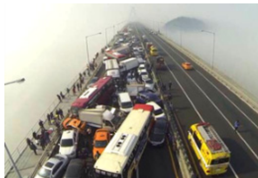
Fig. 1. Accident on Yeongjong Bridge in February 2015.
